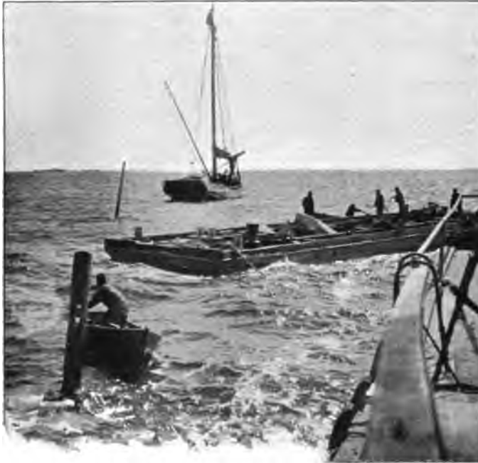
SCOW GETTING INTO POSITION TO DEPOSIT STONE.
